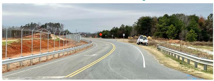
The portion of Old Dowd Road between Marshall Drive and Wallace Neel Road reopened this morning after a two-month closure. During the closure, crews installed a new drainage system and prepared for construction of the fourth parallel runway and associated taxiways.
